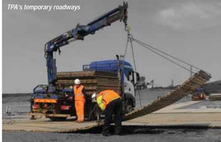
and ground protection plates etc... The company is happy to help solve any ground bearing problem - routine or specific.
